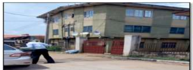
Plate 1.1: Semi-detached three bedrooms flat building, with sliding in ground floor, louvres in first floor and casement in second floor (Field work, 2022).
